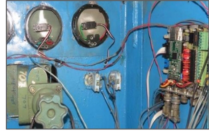
Figure 13 – Servo motors to drive gauges.
